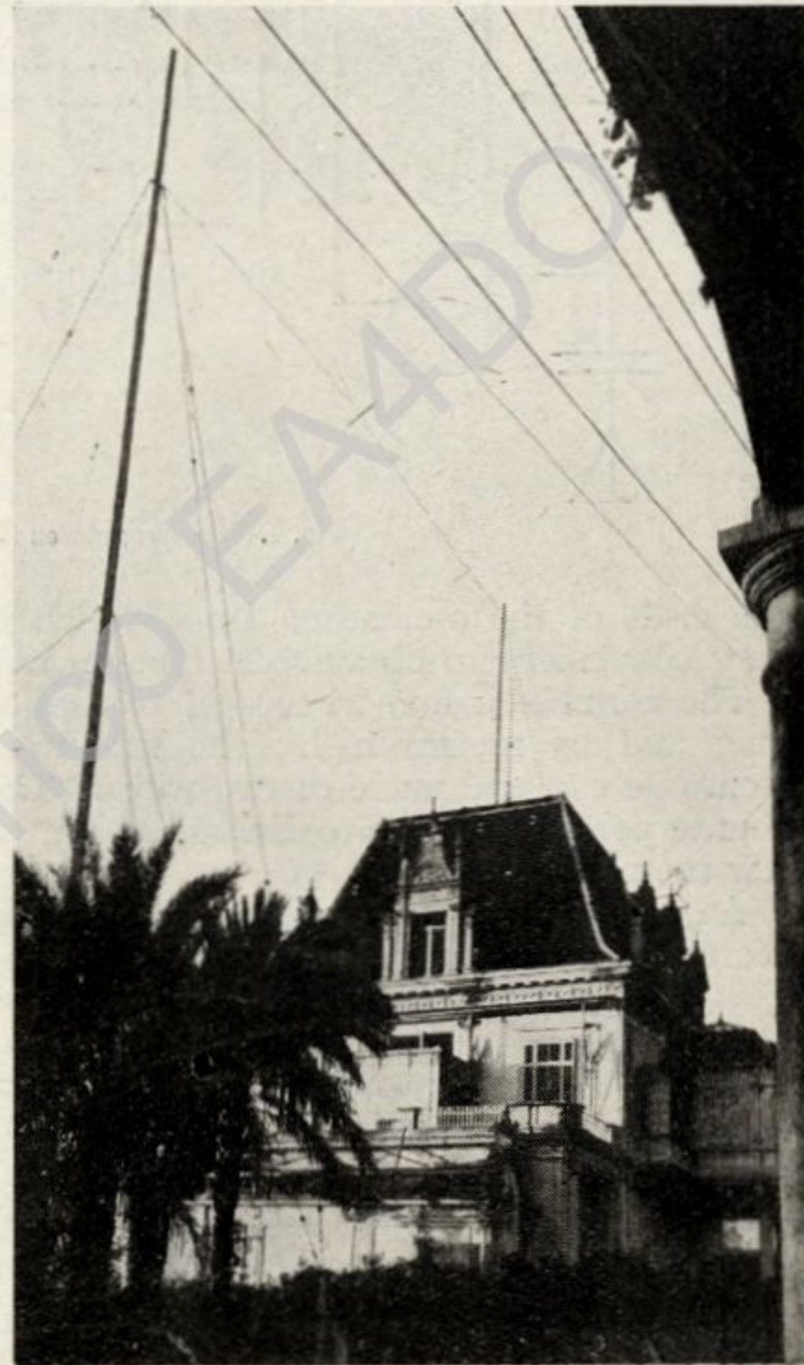
Fig. 3.—Aerial and counterpoise, the far end spreader of the latter being to the right of the palm tree leaves.
